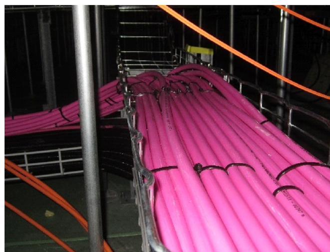
Figure 4 - Cable trays in raised floor
