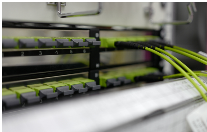
The University of Zurich relies on the tML(standard) cabling system with the 12-fibre MPO in fibre class OM5. Image source: University of Zurich, photographer Teodoro Brasacchio
