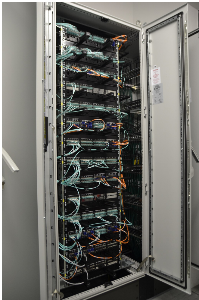
Wintershall Dea uses the modular tML platform with 48 ports, allowing 96 fibres to be used on a single height unit. During implementation, tde took into account older specifications from the former structure of the plant.
