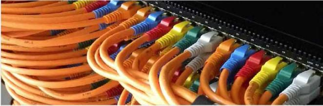
tain challenges: for example, data cabinets are very tightly fitted. 600 cables in one cabinet lead to space problems. Furthermore, the implementation of so many connections takes a long time thereby increasing expenses. The error rate of large cabling projects is also not to be underestimated: If technicians are busy with inserting plugs for hours plugs could be placed in the wrong location.
